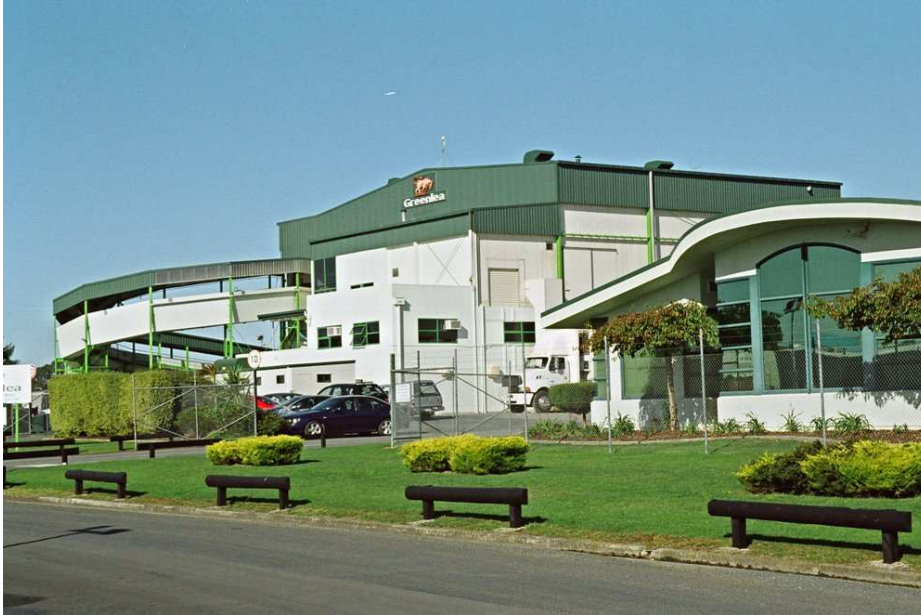
Greenlea Processing Plant, Hamilton, New Zealand
