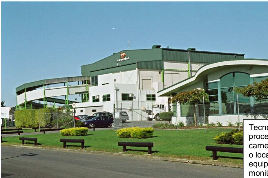
Fabrica de processamento Greenlea, Hamilton, New Zealand
